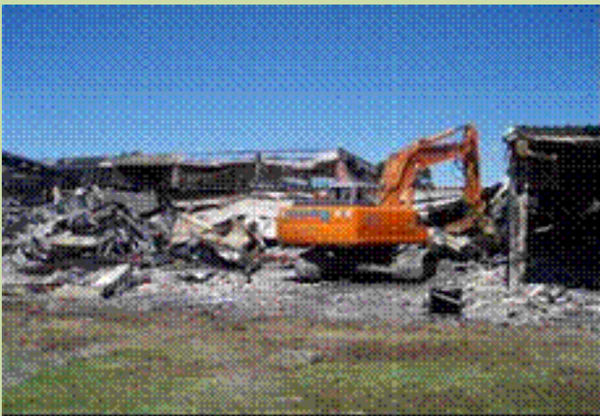
Demolition work following the Bridgewater High School fire in October 2007.
