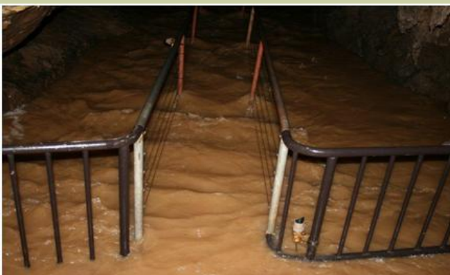
Flood damage caused in the Gunns Plains Caves on the north-west coast.
